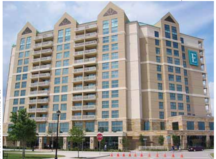
Buildings with large window areas, such as this hotel, require windows with a solar heat gain coefficient, or SHGC, that matches the needs of the climate and the interior environments.
