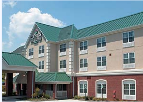
Country Inn & Suites, Knoxville, Tenn., uses single-hung, fixed fiberglass composite windows. Architect: Cope Associates, Inc. Photo: Courtesy of Pella Windows
