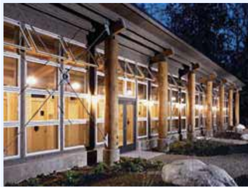
Aluminum-clad wood windows at Island Wood, Bainbridge Island, WA, by Mithun, are positioned for maximum airflow and light.
