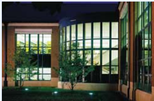
Wayland Union Middle School, Wayland, MI, by Design Plus, Inc., shows how dual glazing with between-the-glass window treatments reduces maintenance.
