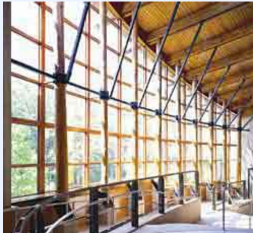
Wood-framed glazing complements the beautiful view of the woodlands at Lakeside Nature Center, Kansas City, MO, by International Architects Atelier.
