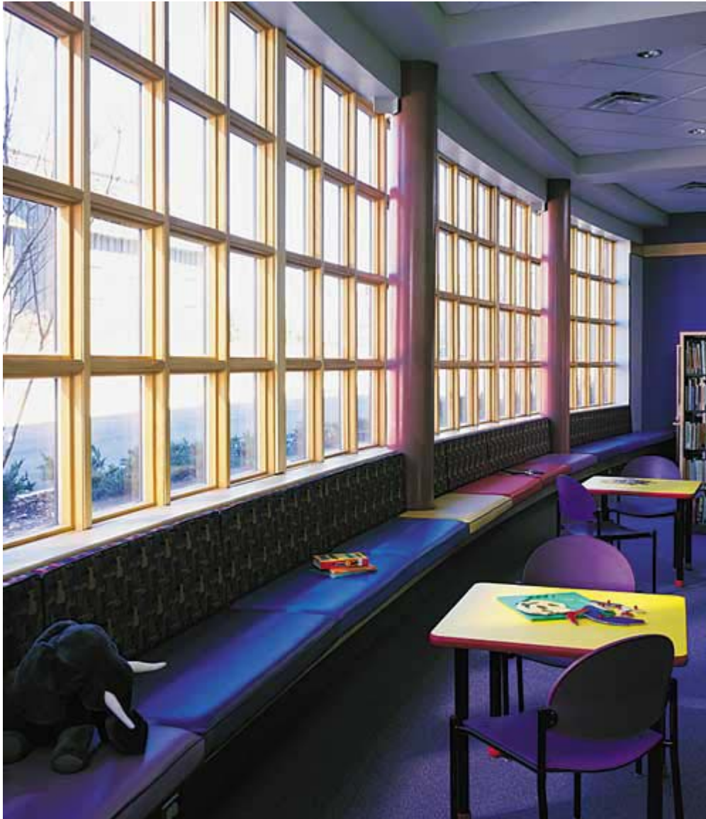
The design team selected individual two foot square wood windows to create a wood grid on the interior that contributes to the warm and natural atmosphere.
