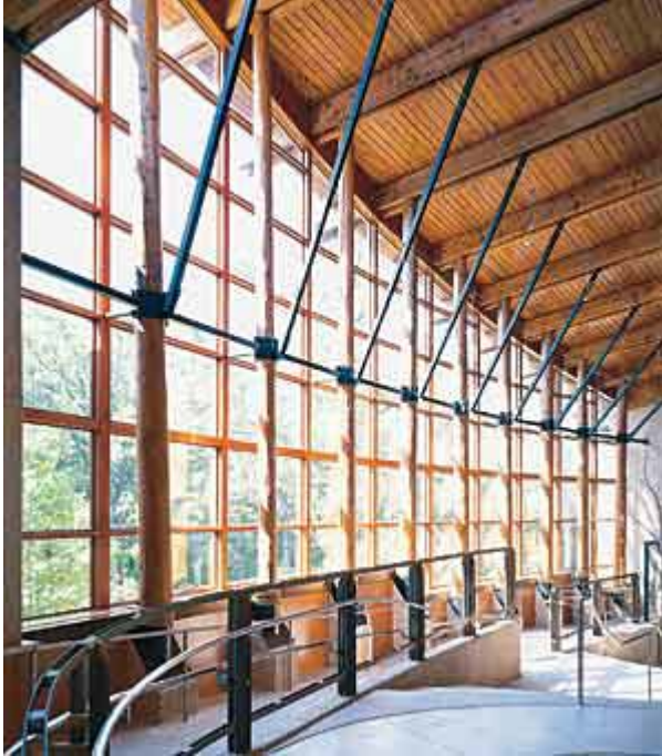
At the Lakeside Nature Center in Kansas City, aluminum-clad wood fixed windows with low-E glass provide a beautifully framed connection to the outdoors while allowing maximum daylight with minimum heat gain. Courtesy of Pella Corporation
