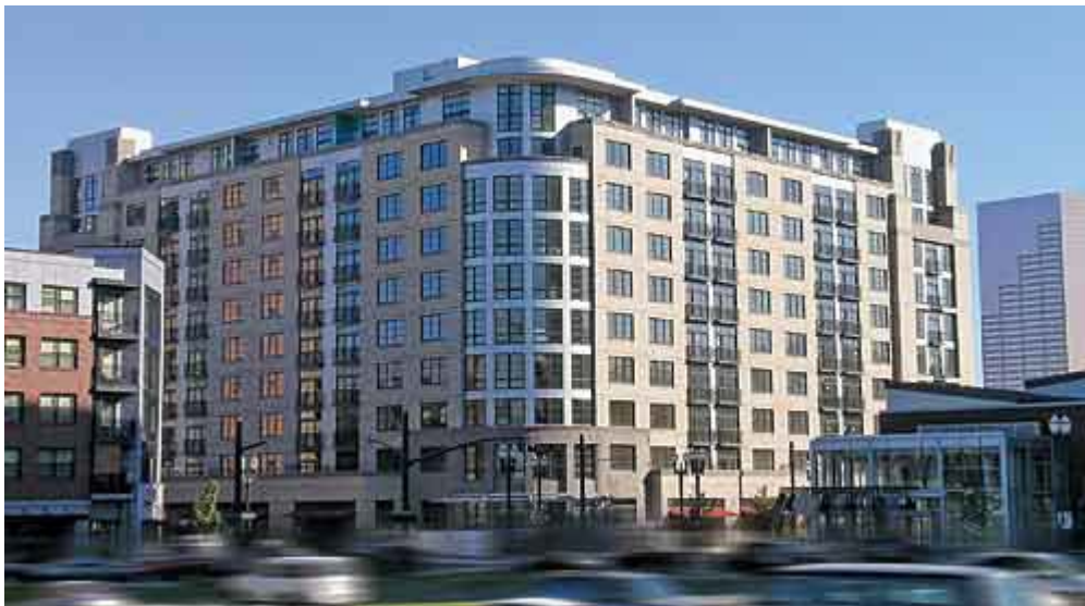
At Burlington apartments in Portland, OR, Ankrom Moisan Associated Architects specified wood windows to meet the developer's energy-efficiency requirements more cost-effectively than aluminum.
